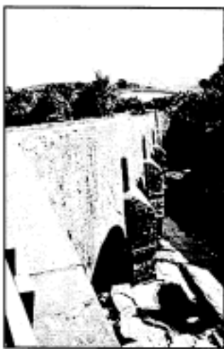
Brynich Aqueduct, Monmouthshire and Brecon Canal prior to work taking place
