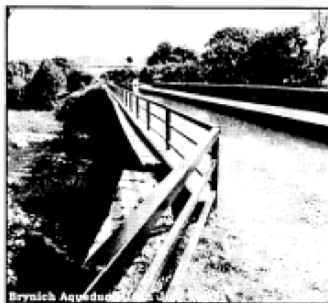
Brynich Aqueduct, following completion of the works in 1997
